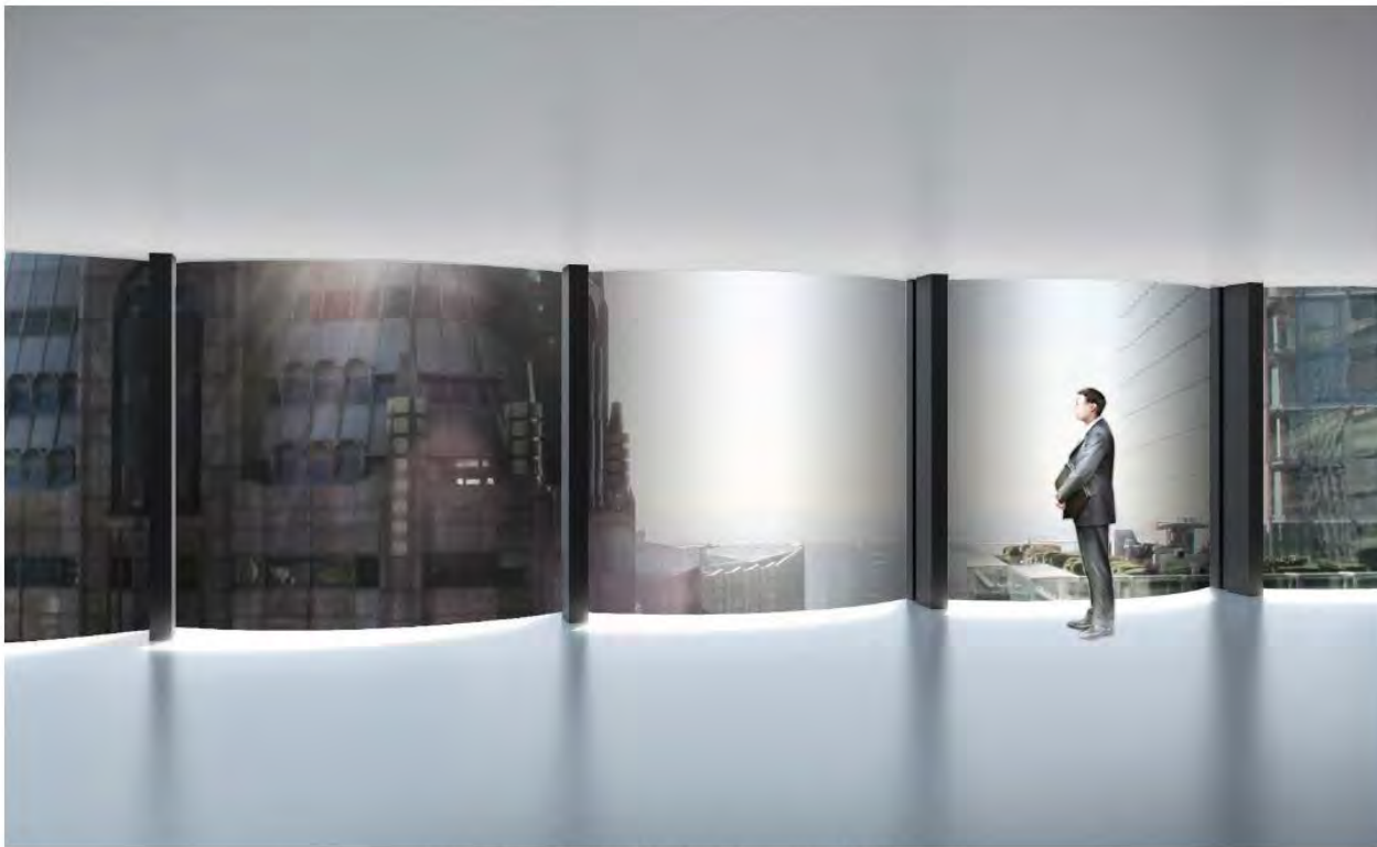
View from interior 3m spacing fluted curtain wall- showing frit gradient effect
